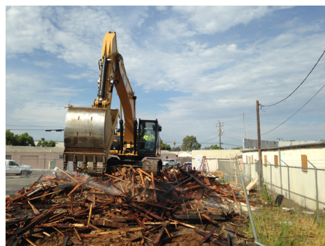
J. Kroeker, Inc. demolishing the Hollywood Inn in downtown Fresno on July 14.
