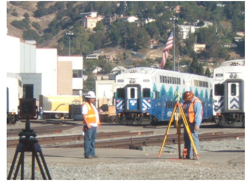
Wagner Engineering & Surveying employees conducting survey work in So Cal.
