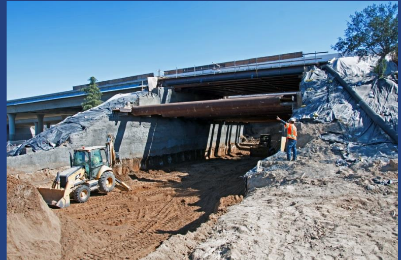
Fresno Trench & State Route 180 Passageway
