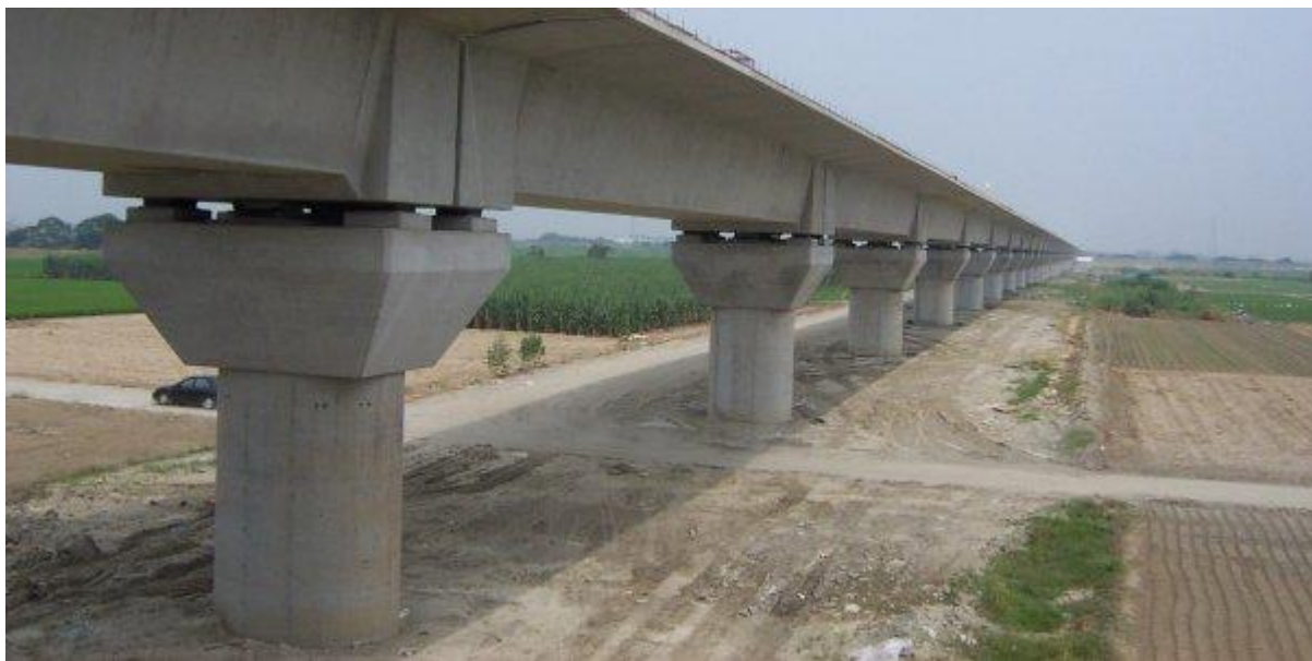
Figure 3-8: Taiwan High-Speed Rail Viaduct
