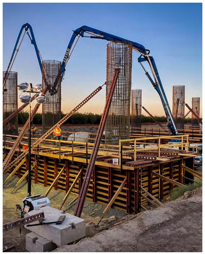
**PHOTO:** Work continues on rebar columns for the Hanford Viaduct.
