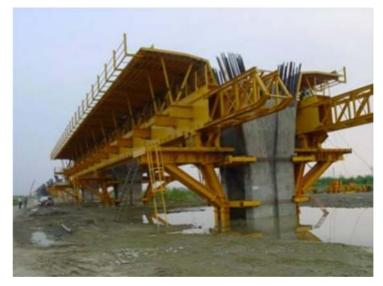
Figure 4-11 Traveling Formwork System from HSR Tech Memo TM 2.3.3 Figure 3-12
