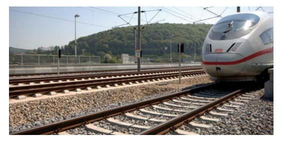
Figure 4-13 Ballast Track - Schotteroberbau
