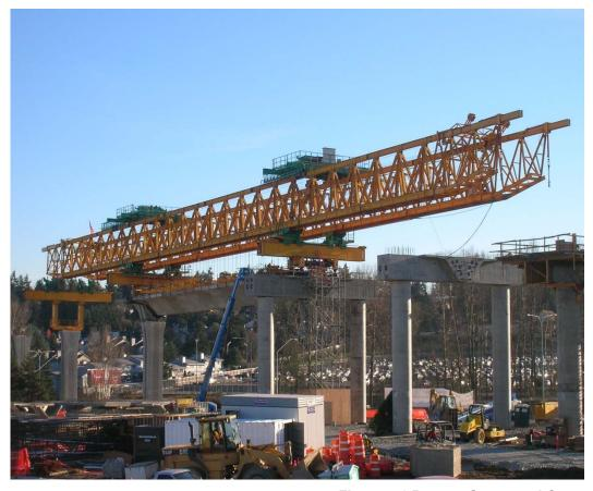
**Figure 4-6 Precast Segmental Construction**
