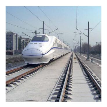
Figure 4-16 Slab Track - China HSR
