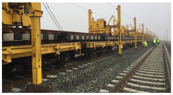
Figure 10. Transportation of a pre-assembled turnout
