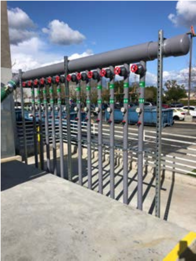
Soil vapor extraction (SVE) system manifold (left) and control panel (right)
