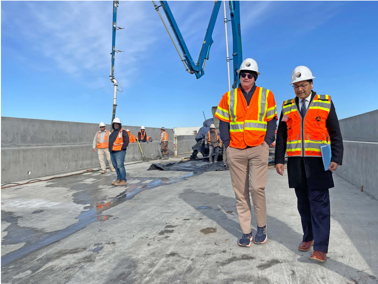
Photo: CEO Brian Kelly and FRA Administrator Amit Bose tour the Cedar Viaduct in Fresno
