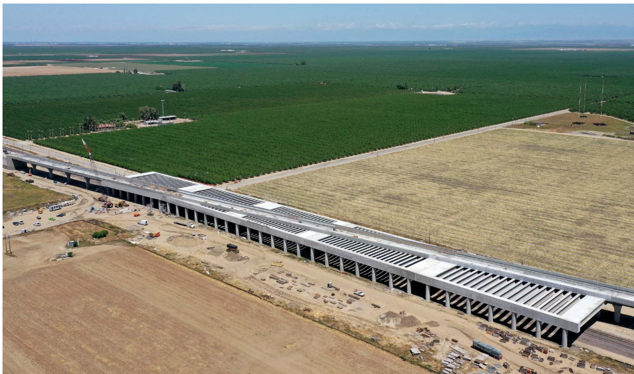
Photo: Wasco Viaduct in Kern County
