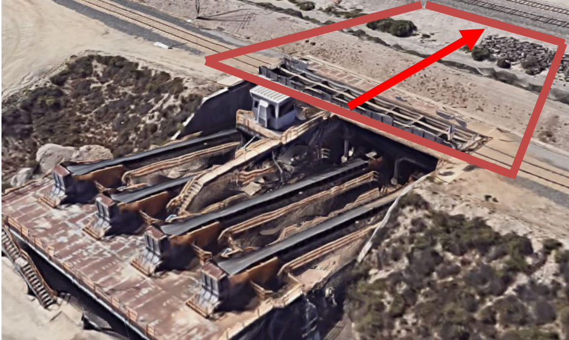
Figure 11-22 Excavation of the New Unloading Pit (Picture of Existing Facility, GE)
