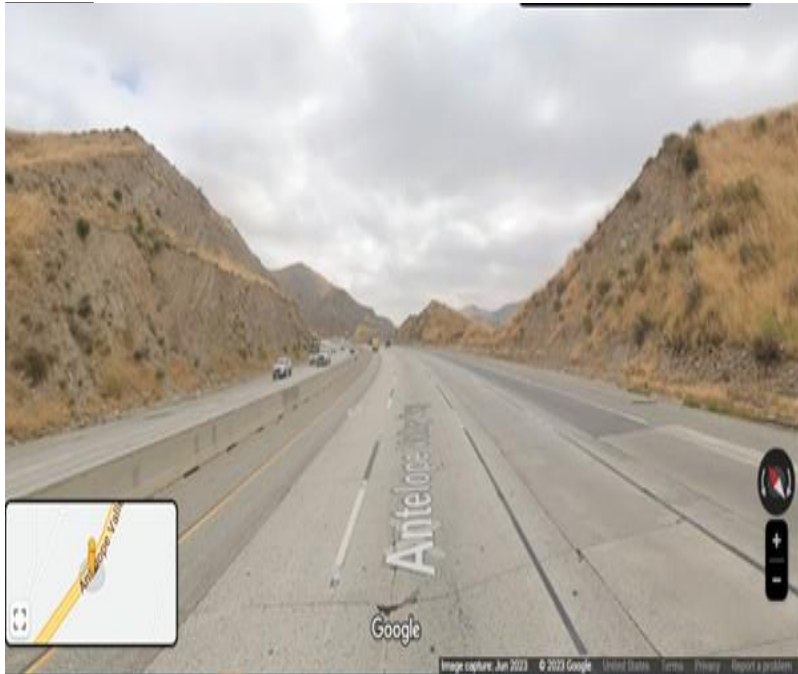
Figure 3. Looking northwest at the steep cut slopes along the SR 14 freeway adjacent to Bee Canyon.
