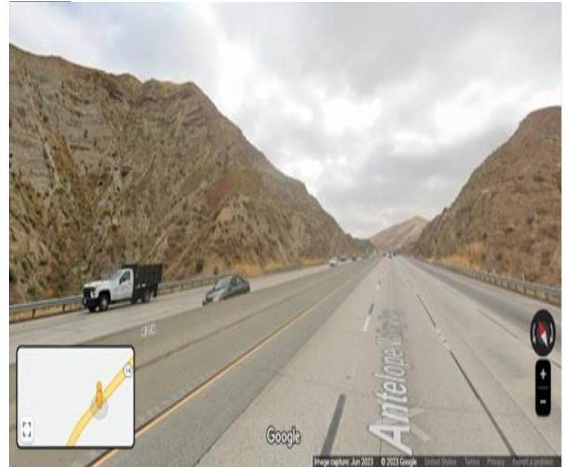
Figure 4. Looking northwest at the steep natural terrain and steep road cuts along the SR 14 freeway adjacent to Bee Canyon.
