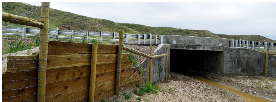
Combined Undercrossing/Drainage Culvert and Wildlife Jump-Out
