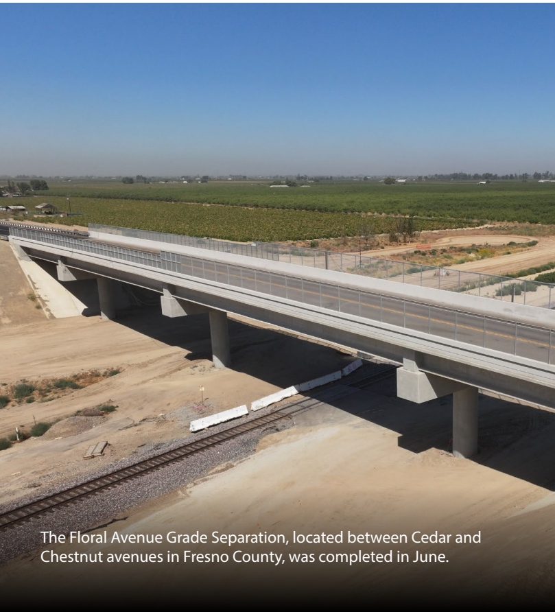
This grade separation is approximately 381 feet long and 40 feet wide. It takes traffic over the existing rail and future high-speed rail lines.
