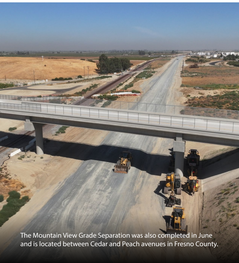
The structure is 368 feet long and 40 feet wide and takes traffic over the BNSF railroad and future high-speed rail tracks.
