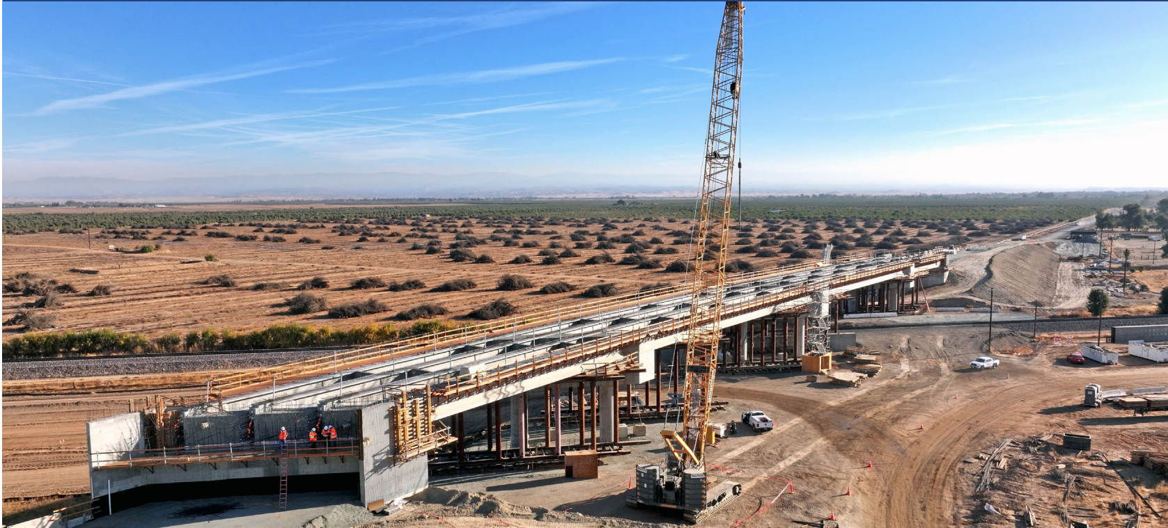
Avenue 17 Grade Separation in Madera County
