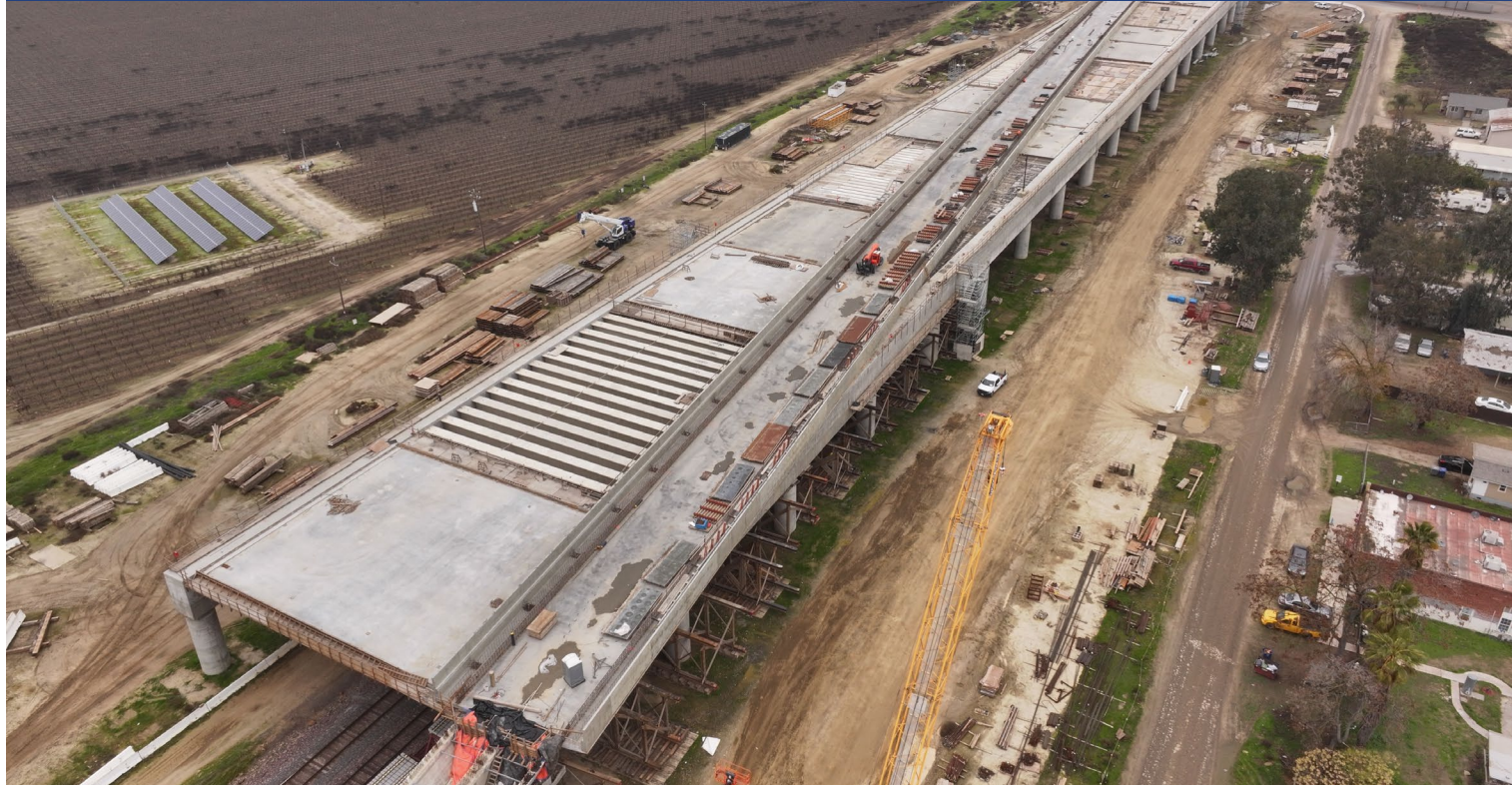
Conejo Viaduct in Fresno County
