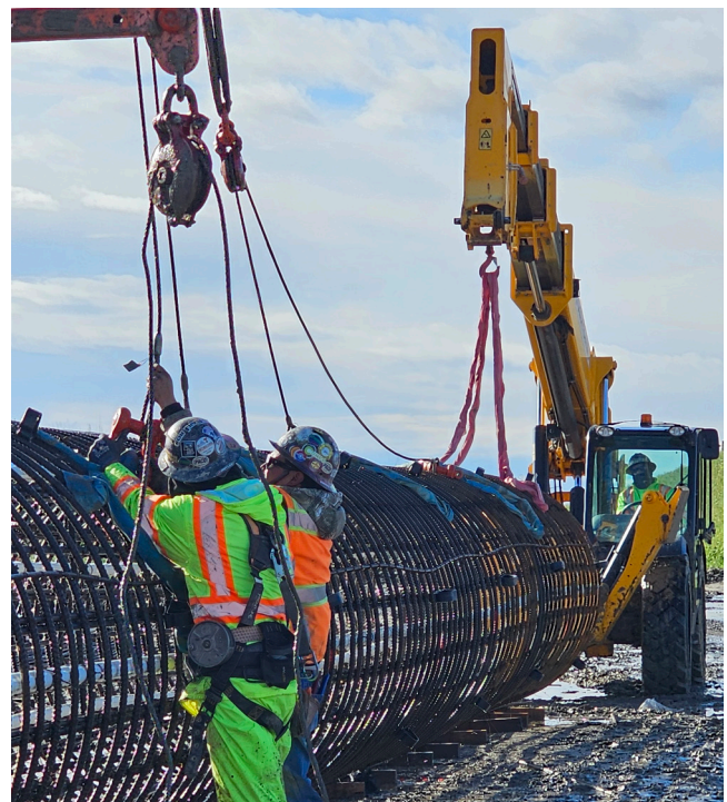
Workers from Mahaffey help prepare a metal rebar tube for placement on a construction site.
