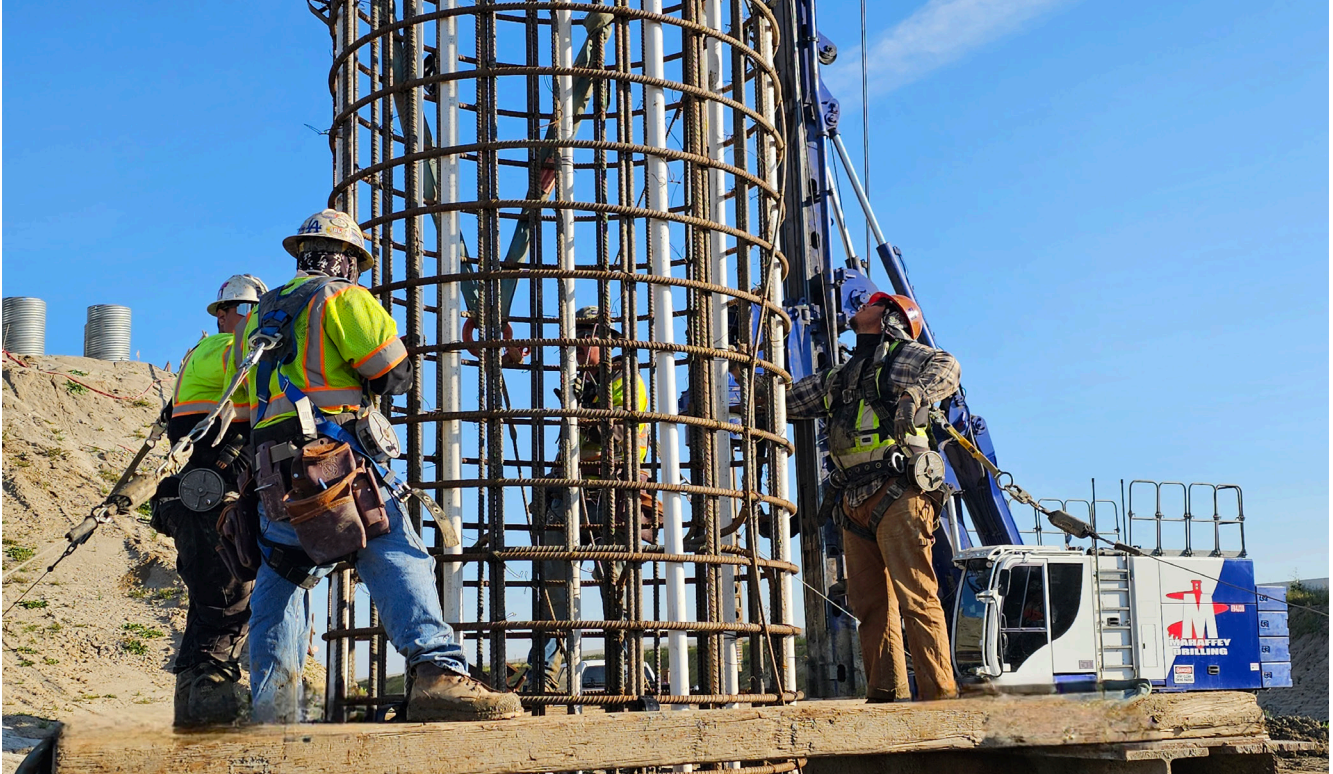
Workers from Mahaffey Drilling work on a metal rebar tube that will help build the foundation of a high-speed rail structure.
