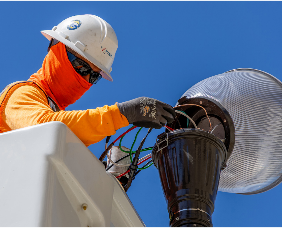
Workers installing the streetlights at the Tulare Street Underpass prior to its completion and opening.
