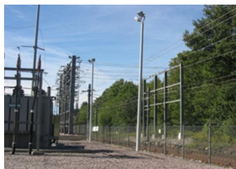
Figure 2-17 Paralleling Station Overhead Contact System Gantry
