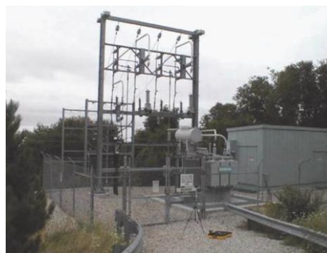
Figure 2-16 Paralleling Station
