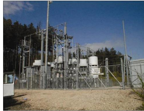
Figure 2-13 Traction Power Substation
