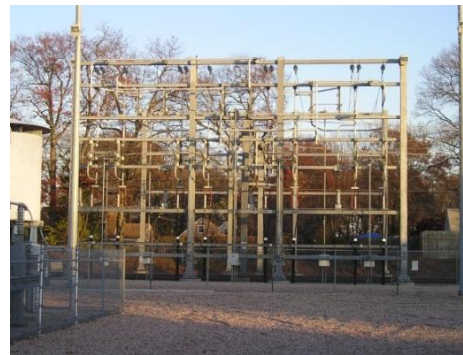
Figure 2-14 Traction Power Substation Overhead Contact System Gantry
