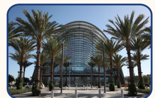
Anaheim Regional Transportation Intermodal Center (ARTIC)
