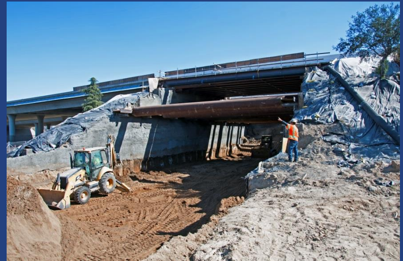
Fresno Trench & State Route 180 Passageway
