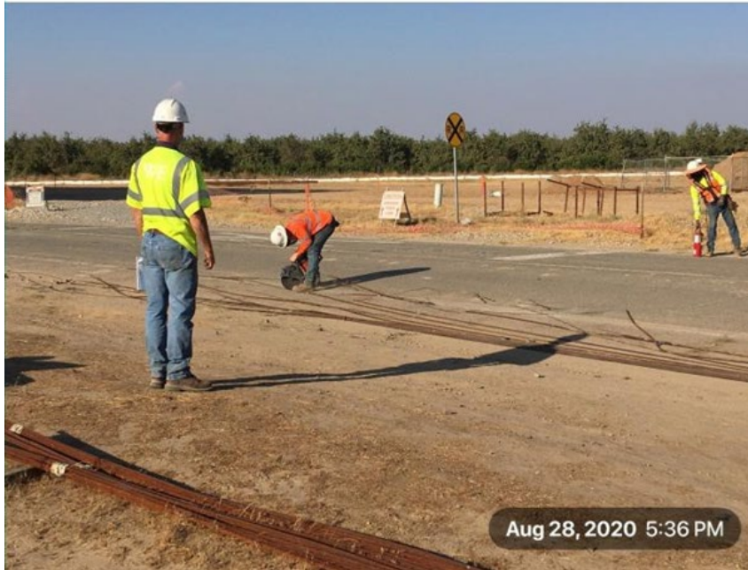
Removal of strands for tagging and inspection from WJE
