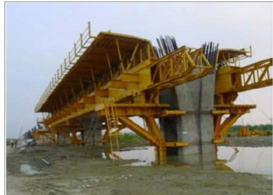
**Figure 2-73 Cast-in-Place Construction on Formwork**
