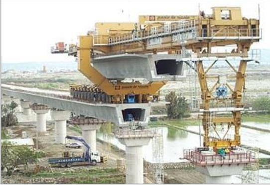
**Figure 2-70 Full-Span Precast Construction on Taiwan HSR**
